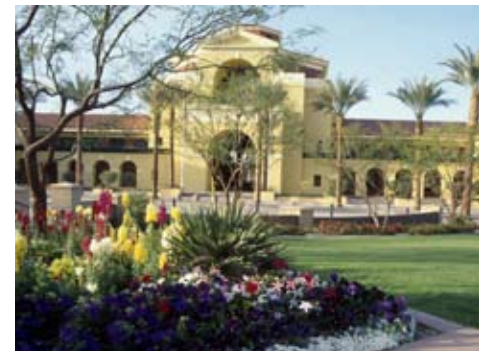
The new City Hall and Town Green provide the first pieces of the new Heart of the City.
