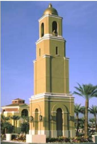
An FTB - designed landmark feature serves as a focal point for the boulevard.
