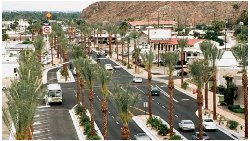
The street configuration along the downtown core segment installed to stimulate desired development; features protected angled parking and slow moving traffic separated from the central fast lanes.
