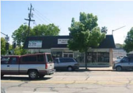
An early challenge was the renovation of an existing First Street 1960's building that housed a thrift store. Its asphalt-shingled mansard and aluminum storefront did not fit the character spelled out in the Specific Plan.
