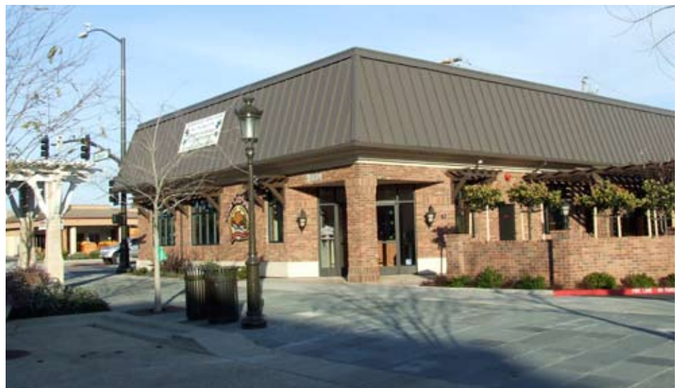
The former thrift store building's completed conversion to a new downtown restaurant incorporating FTS design review input. While the renovation economically re-used the mansard roof (a feature not in keeping with the Specific Plan's preferred roof types), its detailing, materials and color were tied in with its new brick cladding, inset windows, soffit trim and trellis details to fit well with First Street's mix of historic and renovated shops and streetscaping.
