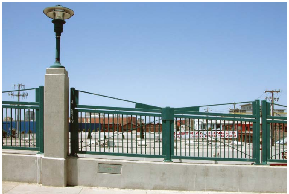
A detailed view of the bridge railing with its diagonal struts and pier-mounted modern lighting fixture.
