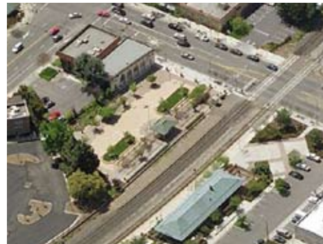
Aerial view of Bill Ball Plaza, ACE tracks, historic Centerville Station, Fremont Boulevard, and surrounding context. The plaza's symmetrical plan is oriented towards future train stop use.
