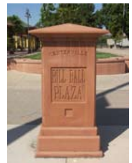
Custom architectural precast concrete pier at Plaza entrance along Fremont Boulevard
