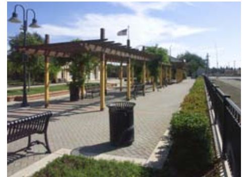
View of Plaza's track frontage with arbor, unit pavers, and plaza furnishings
