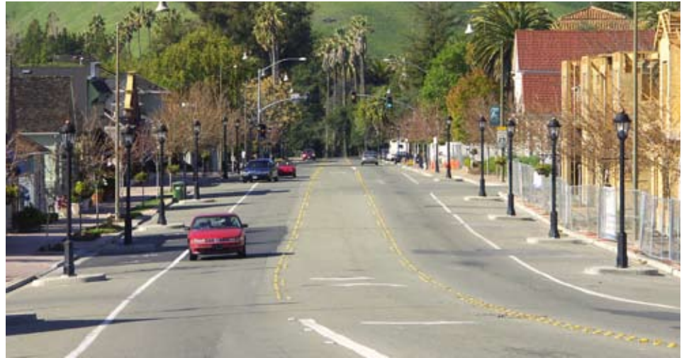
Mission Boulevard’s pedestrian scale was strengthened through placement of new decorative post-top streetlights between parked cars, as well as street trees, benches and other improvements.
