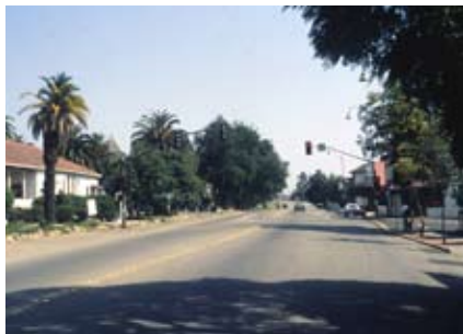
Mission Boulevard’s existing rural charm came with lack of storm drainage and curbs, substandard ADA access and minimal auto-oriented lighting.
