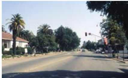
Mission Boulevard had rural charm but lacked curbs, storm drainage, ADA access, and pedestrian-friendly lighting.
