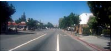
Downtown Livermore before project began.
