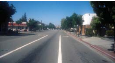
First Street in Downtown Livermore before the project.
