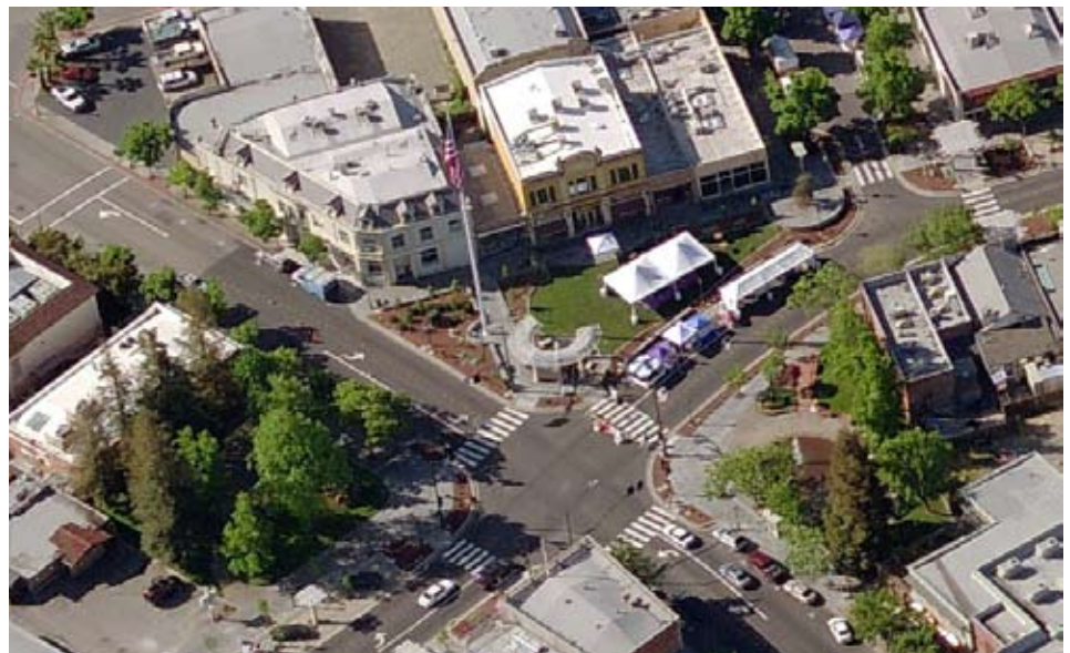
A right-turn "slip lane" was closed and the area it occupied turned into a central town green.
