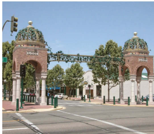
The Downtown Gateway Arch creates a dramatic entrance to the district.
