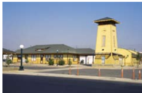
The new clock tower designed by FTB and the adjoining bus station are companion pieces to the restored historic train station
