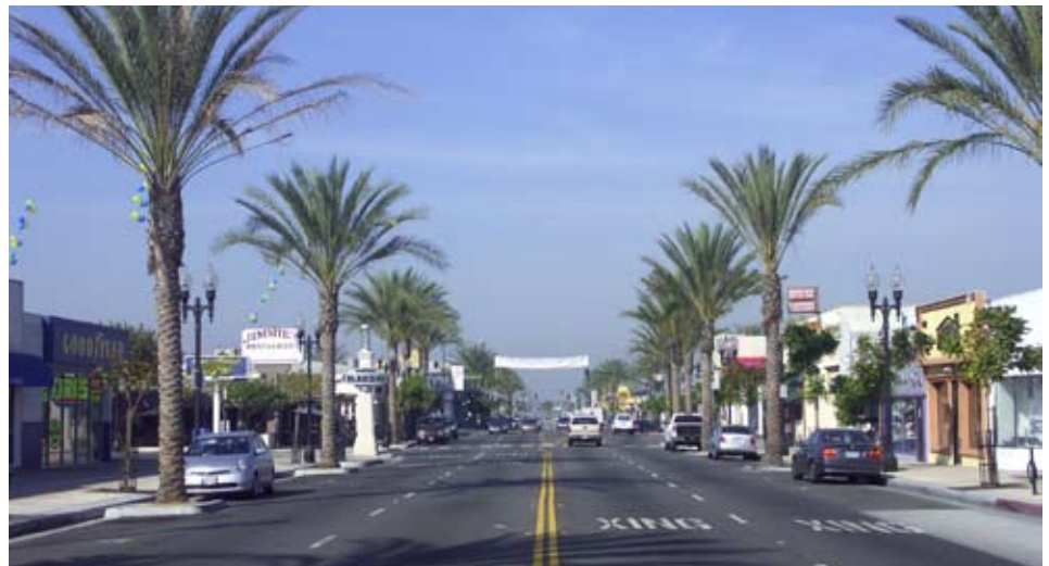
View of the streetscape and landmark improvements completed in 2007. New trees and streetlights are located to visually “narrow” the wide road, strengthen its “grand boulevard” character and enhance pedestrian comfort. Civic sign pylons are used to create gateways and landmarks at special places along the corridor.
