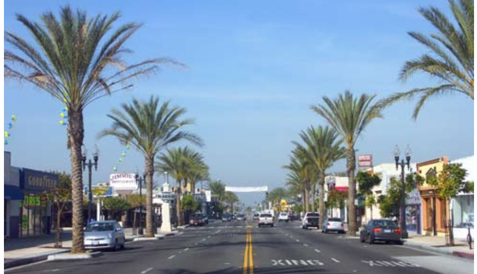
AFTER: View of the completed streetscape and landmark improvements. Trees and streetlights are located and sized to visually "narrow" the wide arterial road, strengthen boulevard character, and enhance pedestrian comfort.
