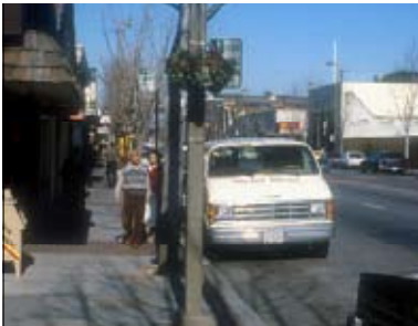
Castro Street's sidewalks were narrow and its roadway was wide and auto-dominated prior to reconstruction.
