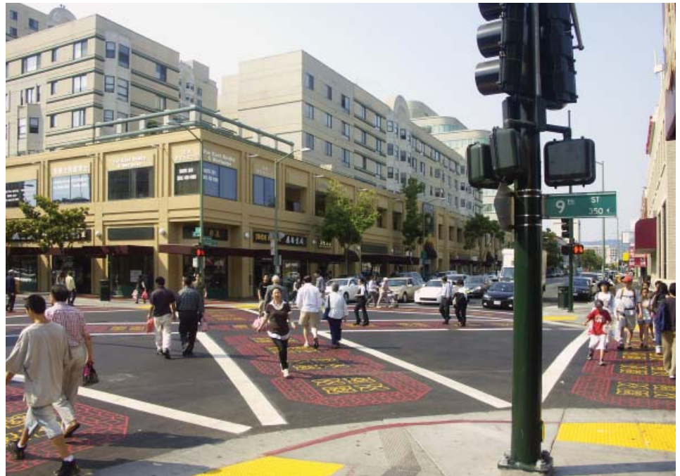
The completed improvements increased waiting room and shortened crossing distances with sidewalk bulb-outs; provided countdown crossing timers and retimed traffic signals; added highly visible and decorative Chinese motifs in the crosswalks; and provided supplementary pedestrian-height streetlights.
