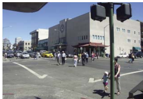
Before: Two experimental "scramble" intersections had long crossings and hard-to-see markings.
