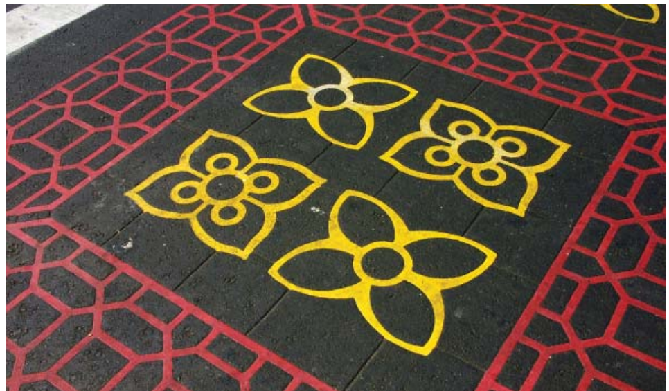
Close-up view of imprinted decorative crosswalk markings, adapted from a Qing Dynasty manual of Imperial Court architectural design and decoration.
