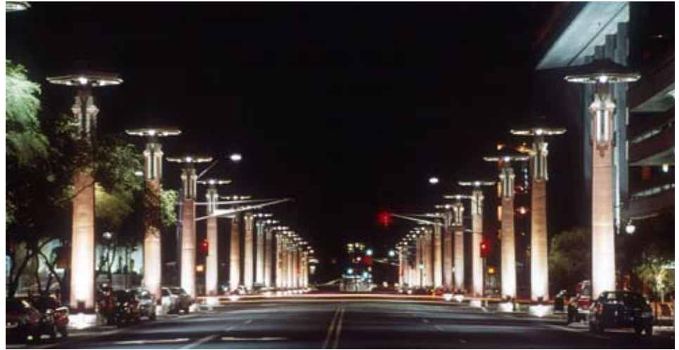
Dramatic "light columns" line Second Street and create a memorable setting for downtown cultural, civic, and sports venues.
