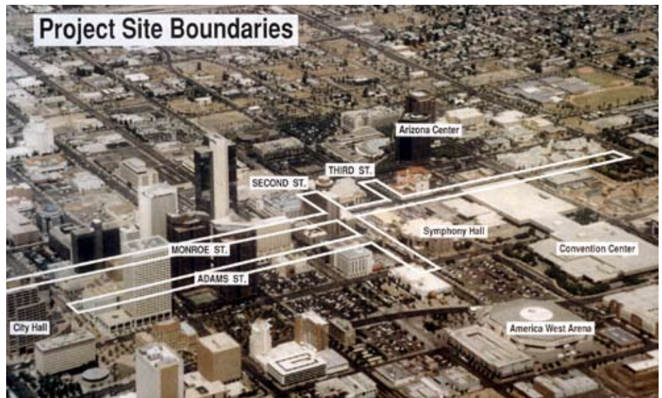
The project area included the three major development corridors in downtown Phoenix. Along these corridors are major convention, sports, and cultural venues and most of downtown's largest office towers and hotels.
