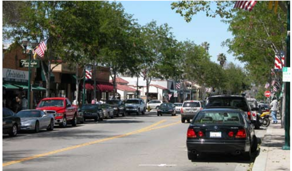
View of Main Street with new streetscape. Purple Robe Locust trees provide shade and seasonal floral color while maintaining views of storefronts. Existing streetlights were repainted to match other furnishings.
