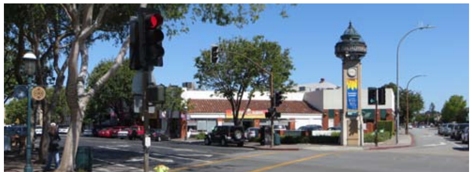
To mark downtown's entrance at El Camino Real, FTB overcame the absence of a memorable building at the "point" of Broadway's angled intersection by positioning a three-sided clock tower with a cylindrical neon-lit "BROADWAY" sign there, topped by an homage to downtown's Courthouse dome. The tower's uplit shaft displays banners for downtown events.
