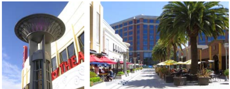
Left: A close-up view of metalwork at the custom-designed lighting columns. Right: An outdoor cafe occupies a portion of the flexible parking/dining area between palm trees alongside the Fox Theatre at right and “On Broadway’s” dining terrace at left.
