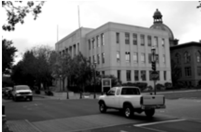
Prior to demolition, a vacant 1939 courthouse annex building covered up the former front of the historic Courthouse at Broadway and Middlefield Road.
