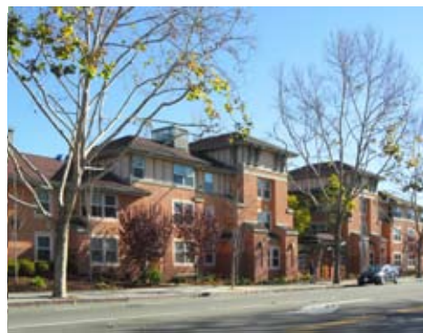
The massing and character of new multi-unit senior housing fit the "Grand Boulevard" setting and were still human-scaled.
