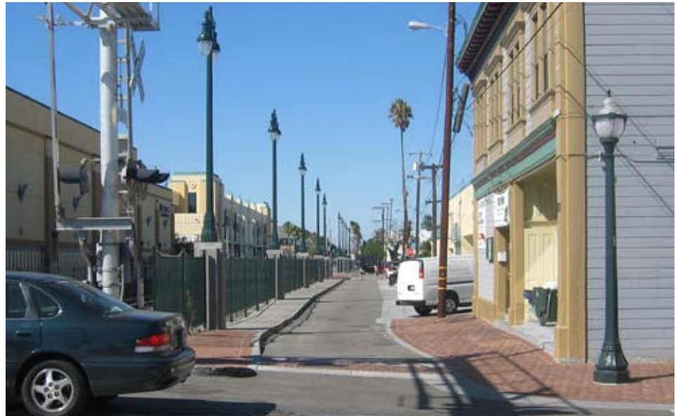
Railroad Avenue after: FTB-designed decorative track edge fencing and a row of pier-mounted twin-head streetlights were installed along with improved paving and brick unit pavers at pedestrian pathways, visible from the adjacent downtown cineplex and nearby public parking structure. The storefront at right has since been renovated into a successful restaurant.
