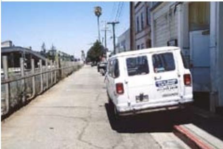
Railroad Avenue before: a service alley with Caltrain edge and fence in disrepair, highly visible from downtown.
