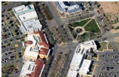
The completed Town Square and Plumas Boulevard spine with surrounding new workplace development.
